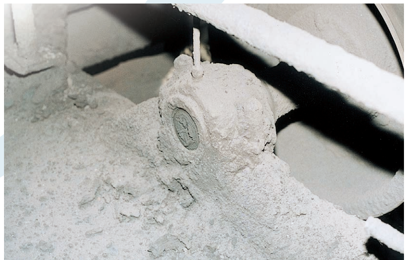
Plummer block usage condition
