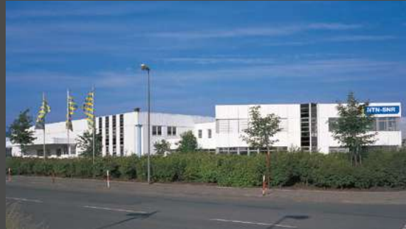
German production facility in Bielefeld
